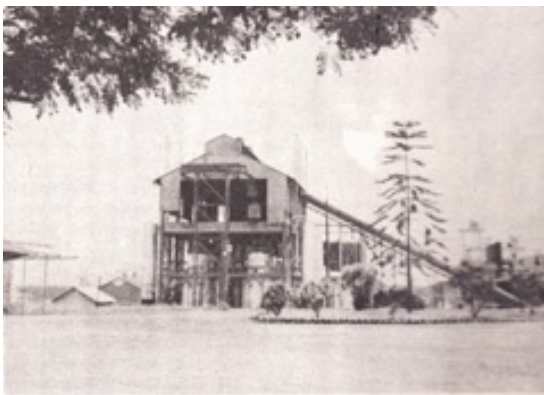
FACT wood gasification plant, the first of its kind in the world
